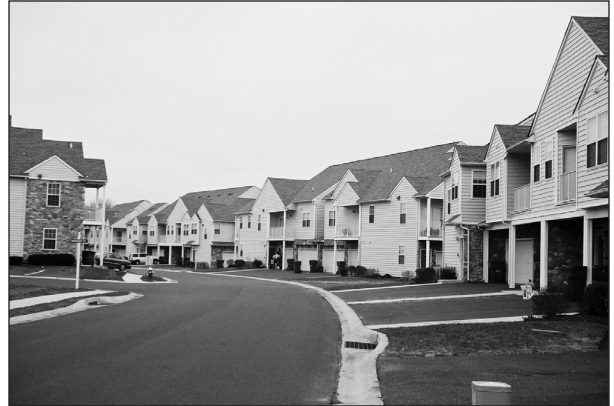
Sadly, this is a street, not an alley.
