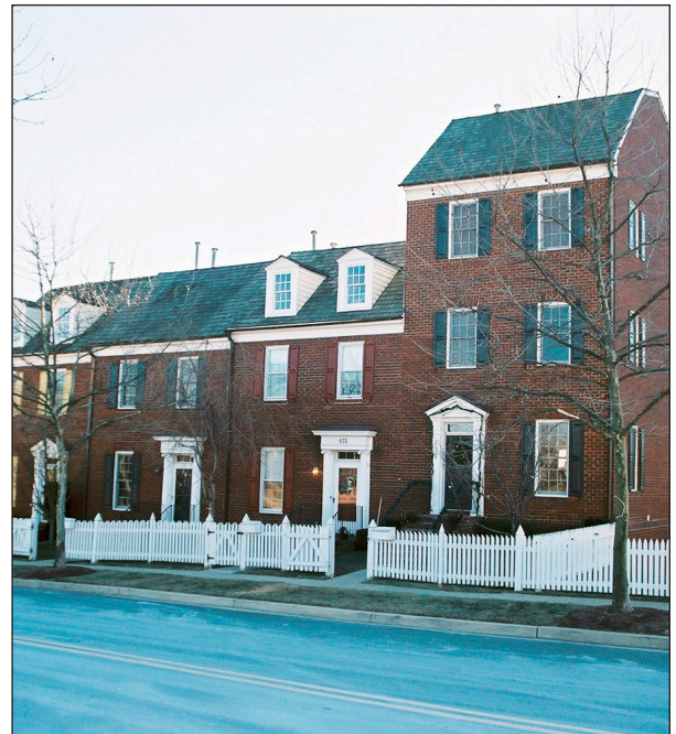
Not all attached dwellings need to look alike - A change in scale and height adds to the vibrancy of a street.
