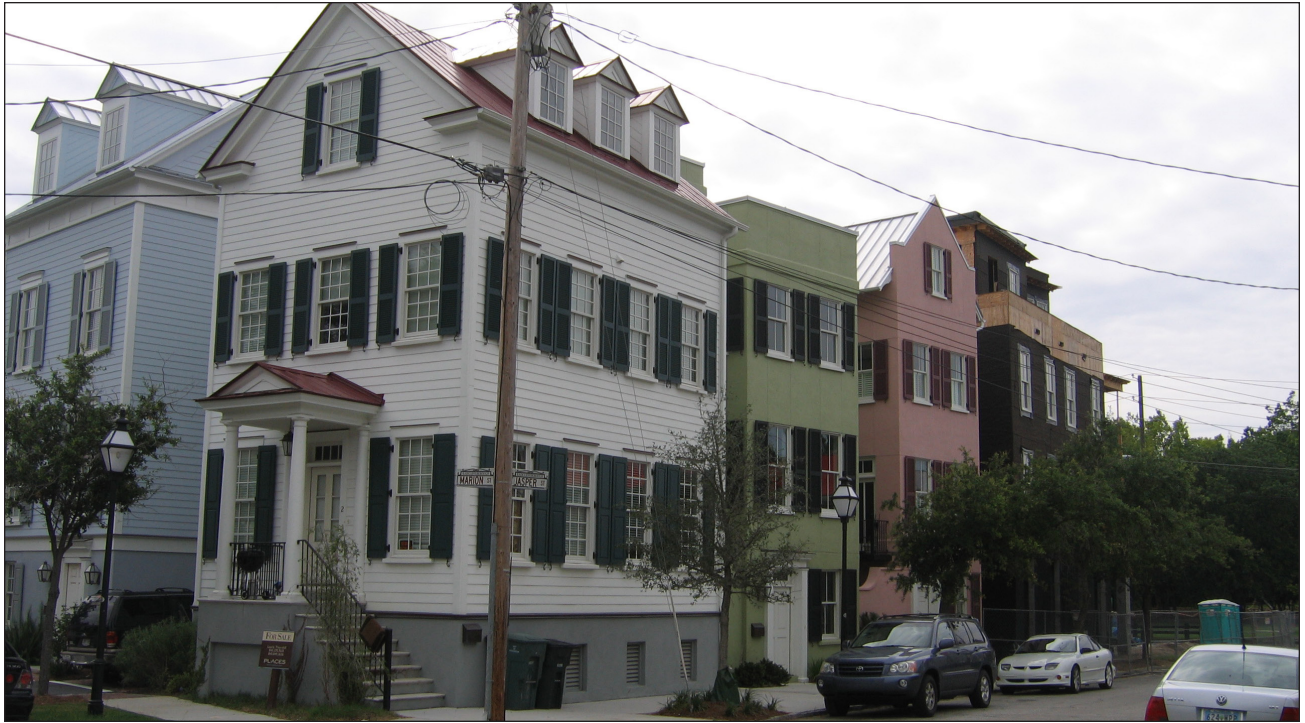
These attached units are broken up by a subtle setback in facade, as well as, differences in material, color, style and contrasting roof lines.
